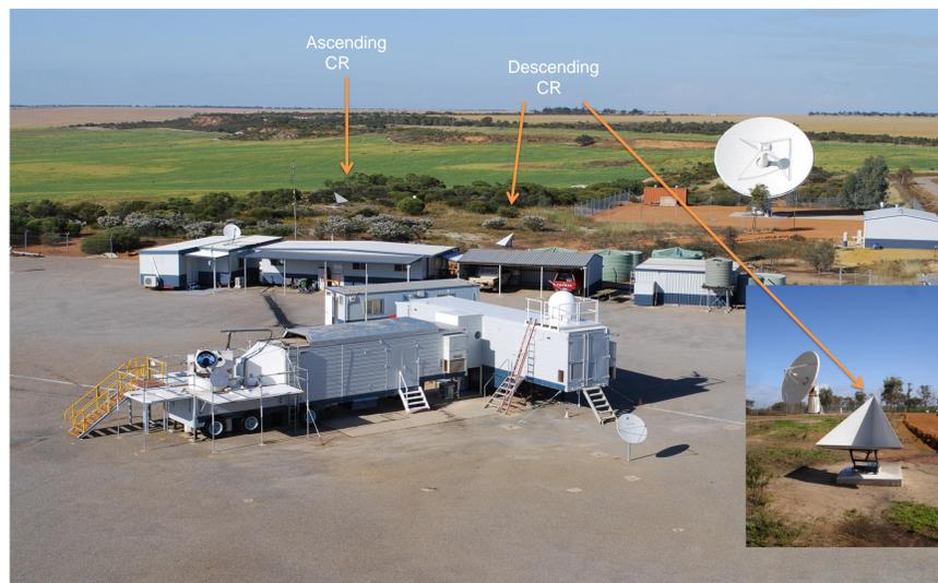
Figure # 2 Site Layout showing new SAR Corner Reflectors
